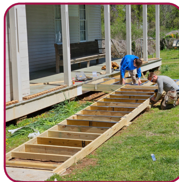
Contractors install the new wheelchair ramp to the Wheeler home porch.
