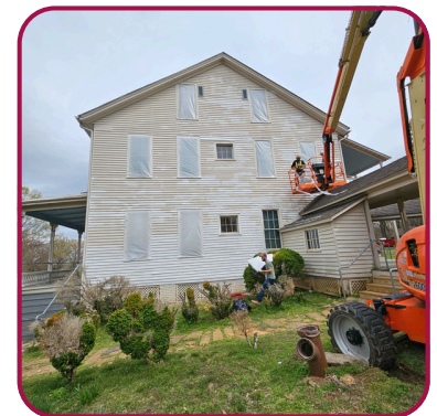
Contractors prep Wheeler Home for exterior paint.
